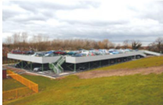
Fast Park® system is wholly demountable and, when removed, will leave no environmental footprint. The asset can be relocated and reassembled at another location and in different configurations.
